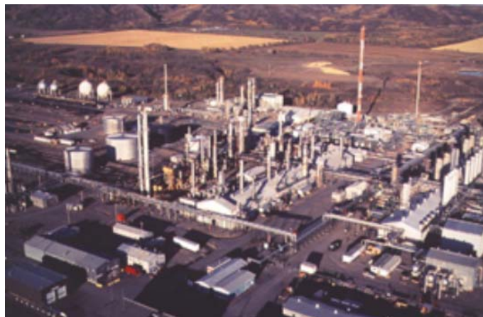
Figure 6- Gas refinery for producing natural gas product.
